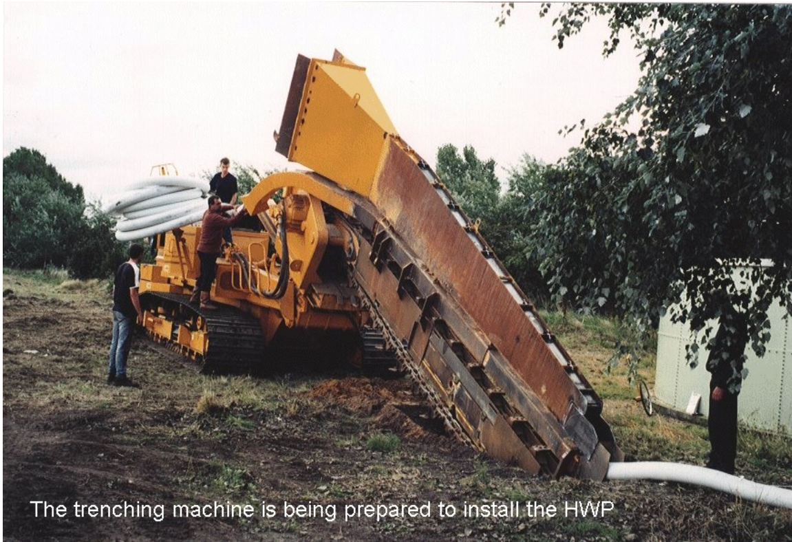
Fig 5 The deep trenching machine ready to start installation
