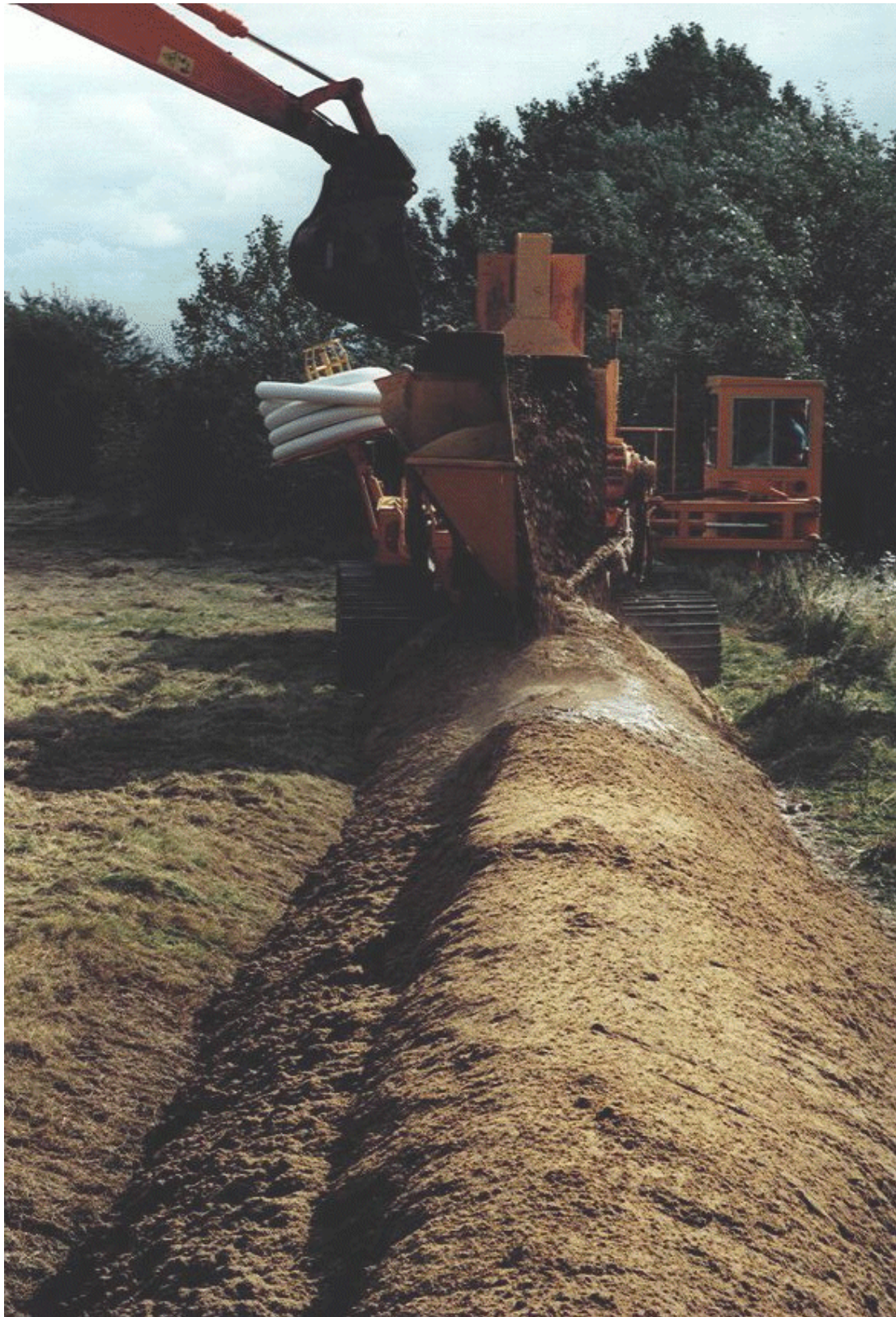
Fig. 8. The trench is being excavated to 6m depth. The wet sand spoil forms a lateral mound along the centre line of the trench and the original ground surface sags with lateral tension cracks running along each side about 1.5 m from the centre of the trench. Once the pipe installation had been completed, the mound was flattened filling the collapse feature.
