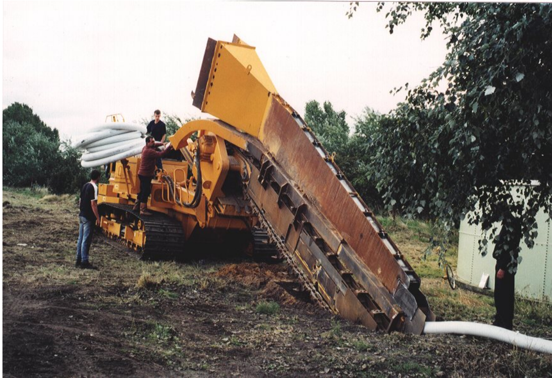
Fig. 7. The trenching machine is seen as the cutting head is being positioned to commence the installation of the horizontal wellpoint with the digging boom fully extended. The continuous chain of buckets runs along the bottom of the boom with the square-section pipe feed-tube immediately above the buckets. Operators can be seen feeding the drainpipe into the funnel on the top of this feed-tube. A second, larger guide-tube lies on top of the assembly to feed filter sand on top of the pipe as it is guided into the bottom of the trench. The filter sand is stored in the large hopper at the top of this feed-tube. The initial length of unperforated drainpipe can be seen extending out of the bottom of the digging boom assembly and has been secured to a stake (out of shot) so that it remains at the surface at the pump end of the horizontal wellpoint. The suction pump was installed at this end of the pipe with water pumped into the adjacent storage tank on the right of the picture.
