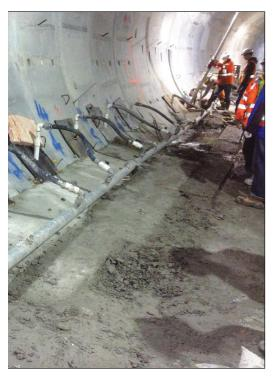
dewatering measures drilled from surface for tunnel construction.
