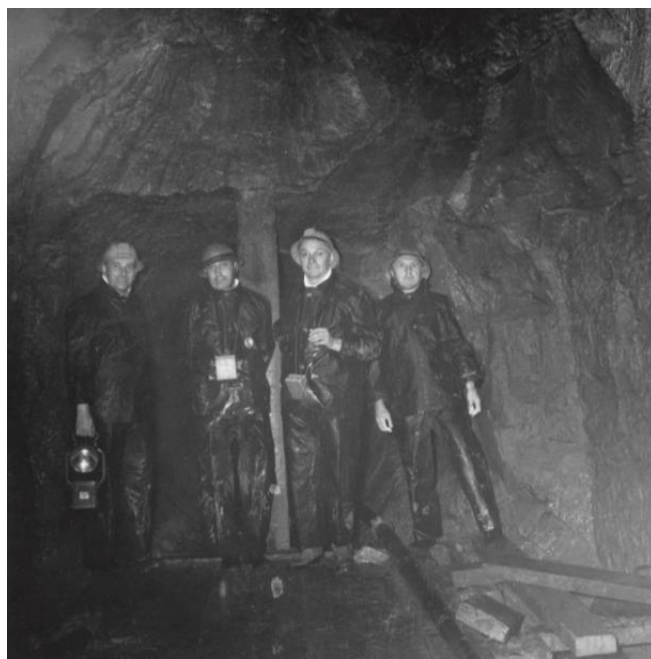
Figure 1. CTSG visit to inspect drained Sangatte Workings, 1958 (courtesy of Amanda Davey).
