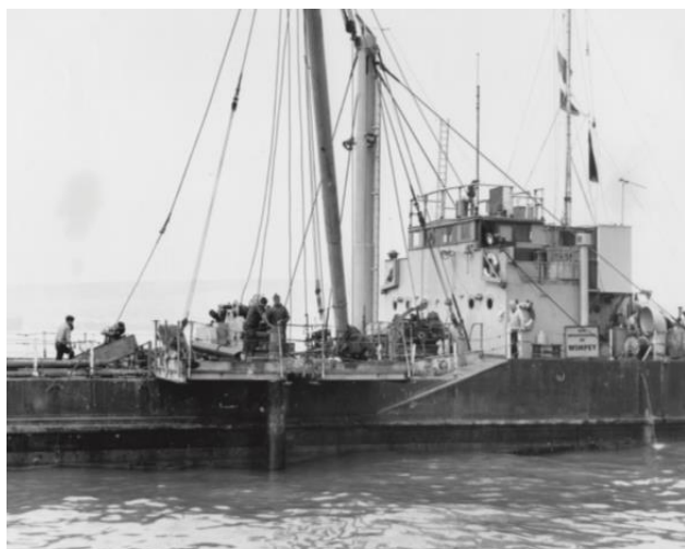
Figure 2. Drilling rig working from platform extended over side of drilling vessel GW14 during 1964–5 investigation (courtesy of Amanda Davey).
